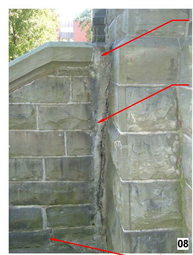
REPAIR CRACK IN STONE (STONE RESTORATION PACKAGE) CLEAN STAINED STONE (STONE RESTORATION PACKAGE)
