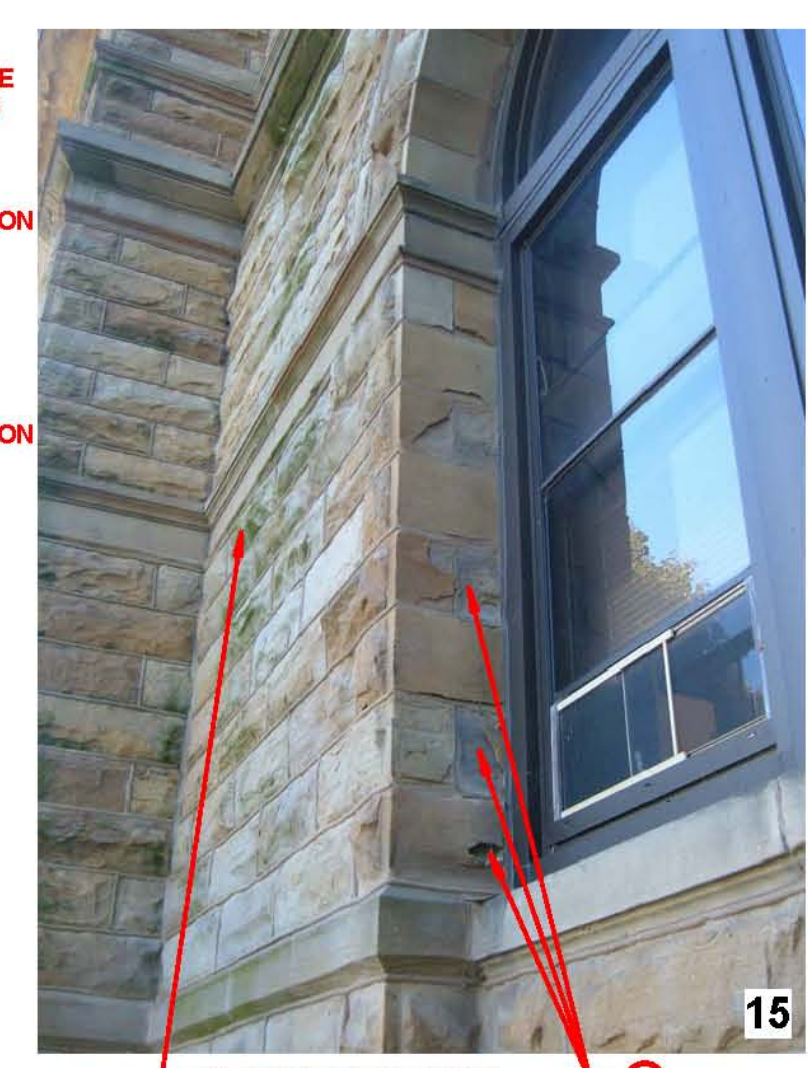
CLEAN STAINED STONE (STONE RESTORATION PACKAGE)
