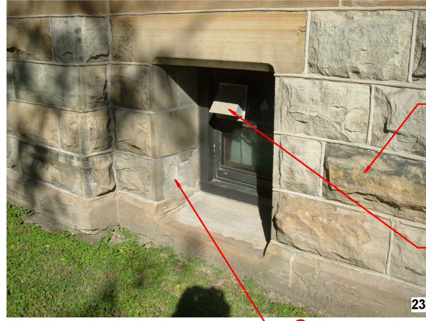
19 REMOVE BOLT, PATCH HOLE (STONE RESTORATION PACKAGE)
