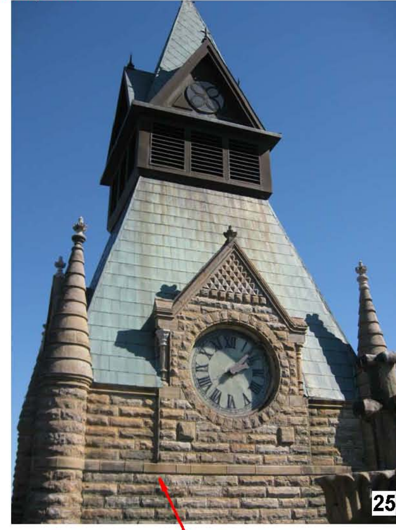
25 CLEAN STAINED STONE (STONE RESTORATION PACKAGE)
