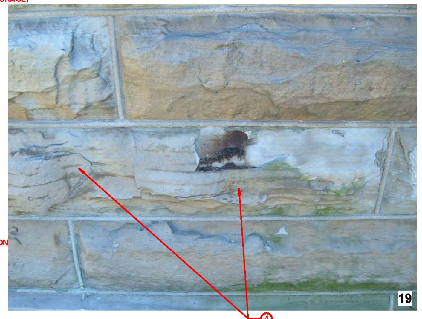
REPAIR JOINT @ FOUNDATION - REMOVE LOOSE MORTAR, TUCKPOINT W/ MORTAR, TYPICAL FOR PERIMETER OF BUILDING. (STONE RESTORATION PACKAGE)
