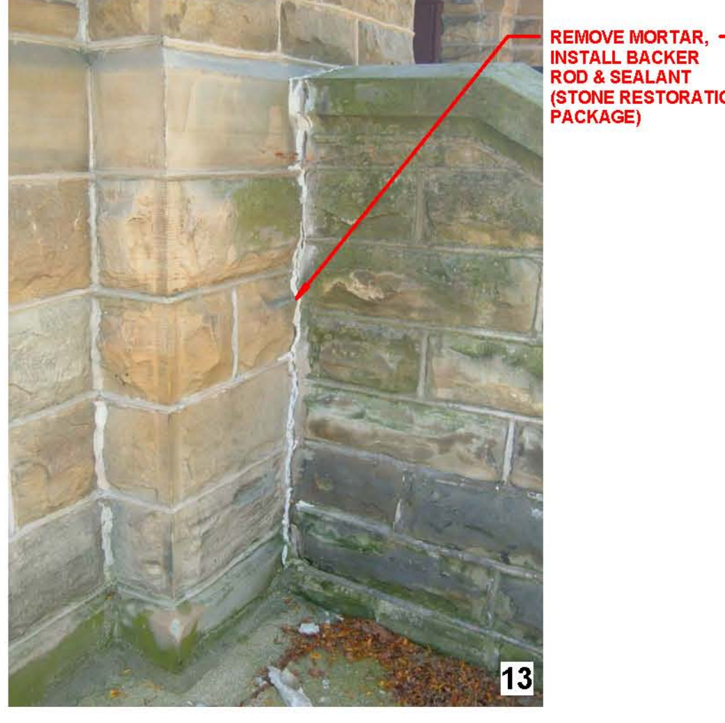
INSTALL BACKER ROD & SEALANT, TYPICAL @ ALL STEPS (STONE RESTORATION PACKAGE)
