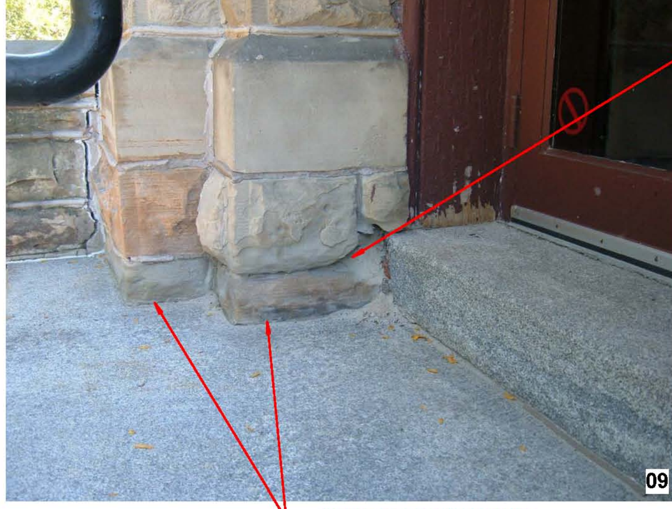
INSTALL BACKER ROD & SEALANT, TYPICAL @ ALL STEPS (STONE RESTORATION PACKAGE)
