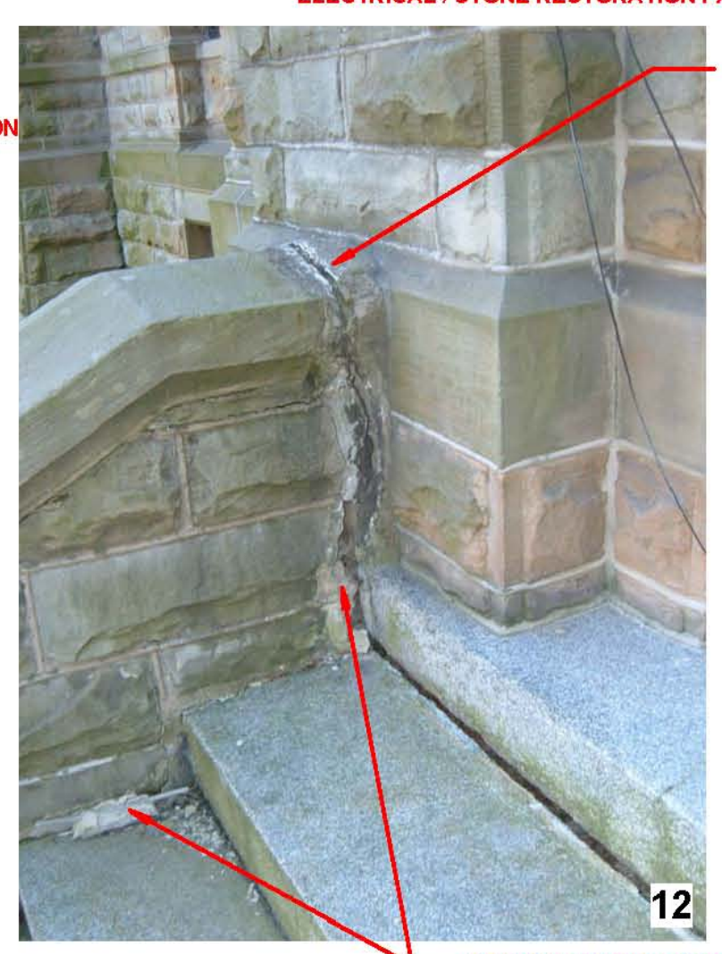
REMOVE MORTAR, INSTALL BACKER ROD & SEALANT. (STONE RESTORATION PACKAGE)
