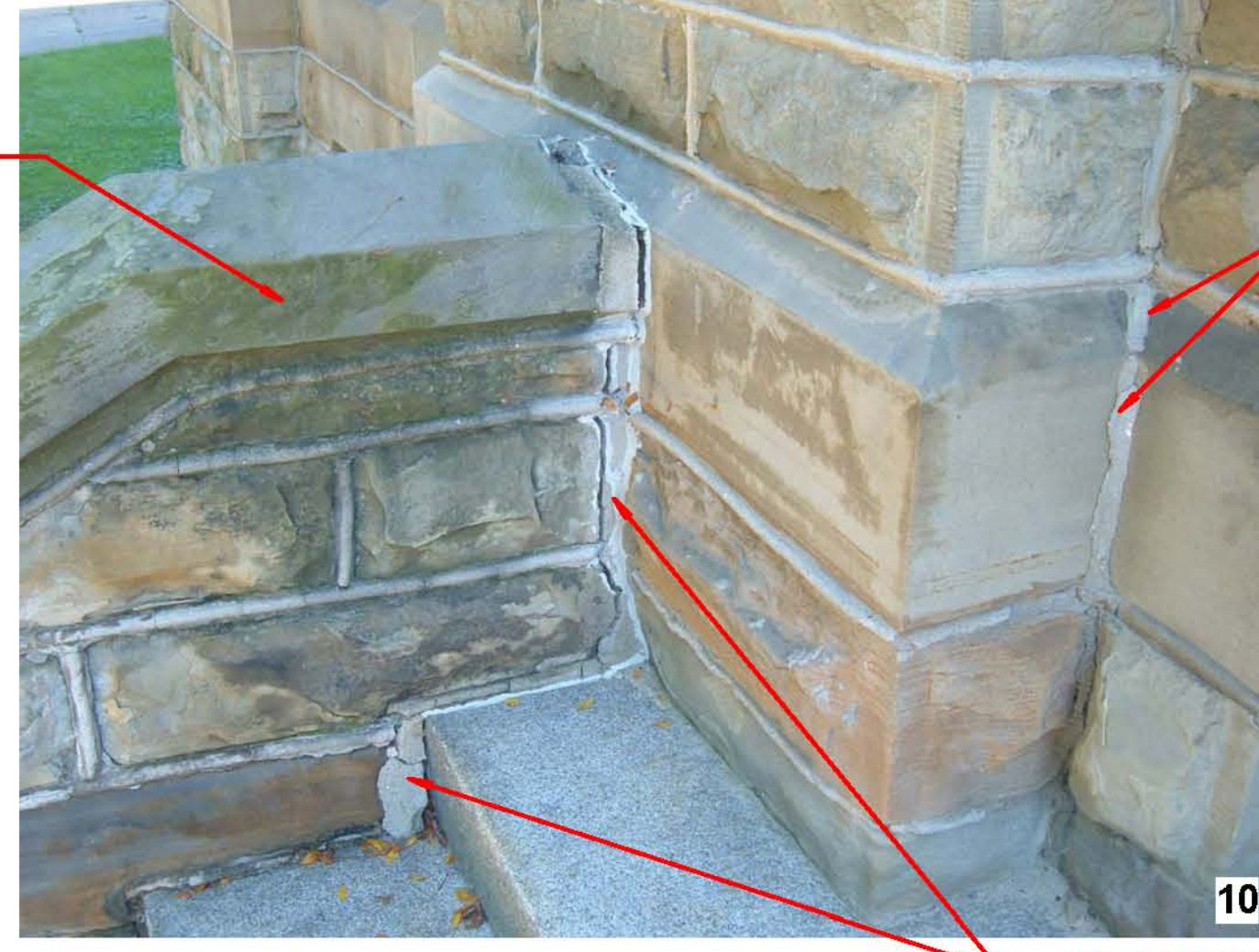
INSTALL BACKER ROD & SEALANT, TYPICAL @ ALL STEPS.
