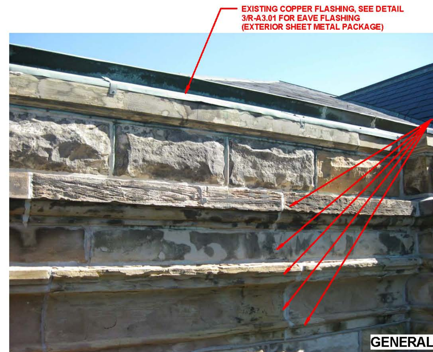
TYPICAL CONDITION OF CORNICE TO BE REPAIRED
