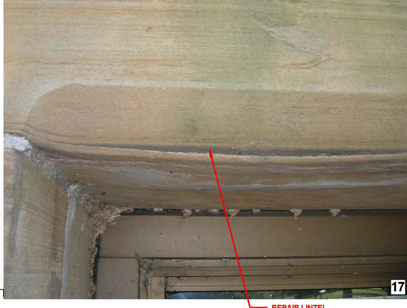
REPAIR LINTEL (STONE RESTORATION PACKAGE)
