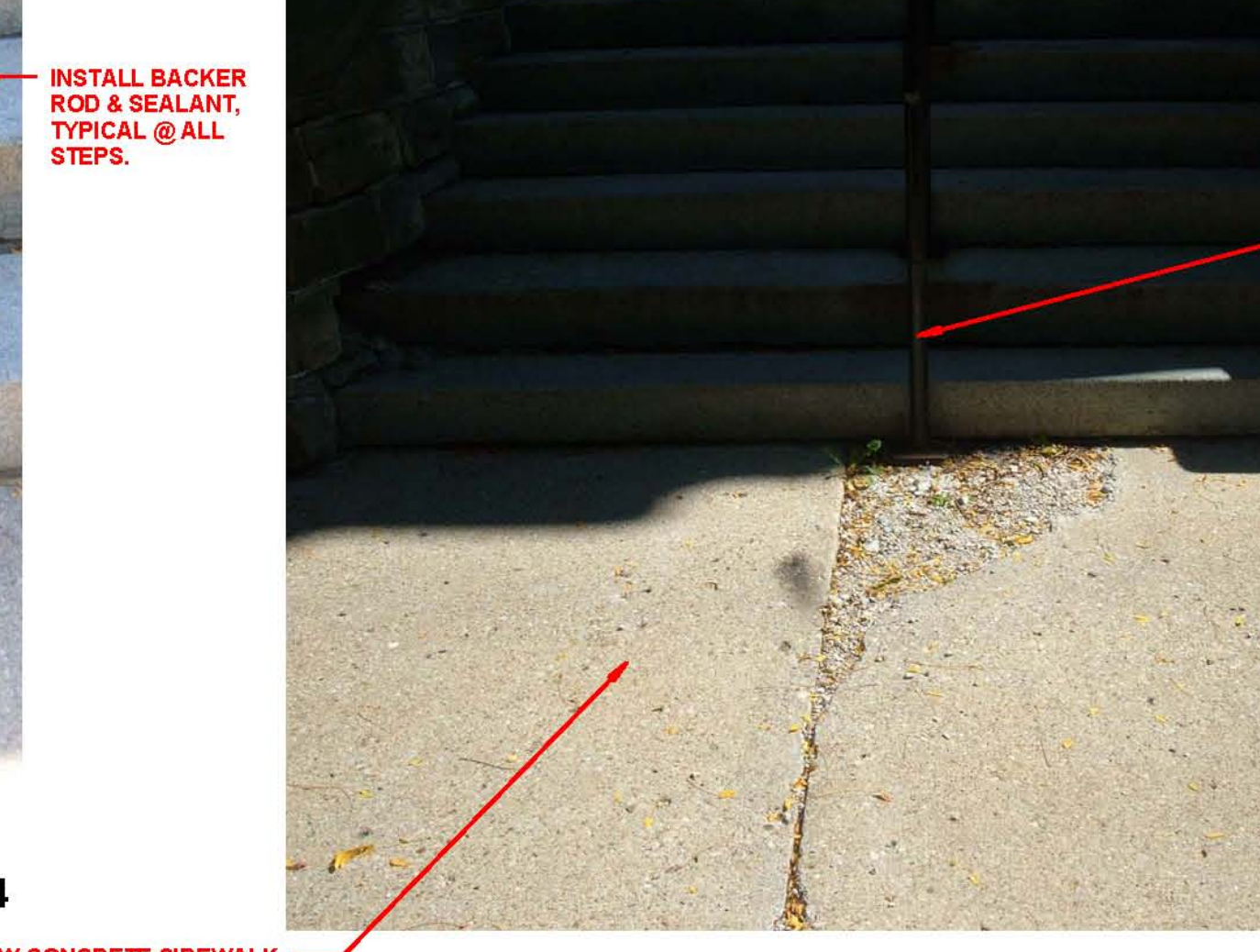
REMOVE MORTAR, INSTALL BACKER ROD & SEALANT, TYPICAL @ ALL STEPS (STONE RESTORATION PACKAGE)
