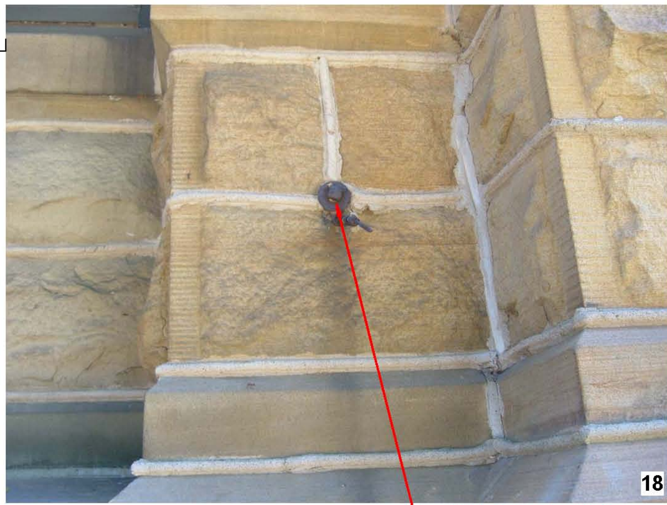
18 REMOVE BOLT, PATCH HOLE (STONE RESTORATION PACKAGE)
