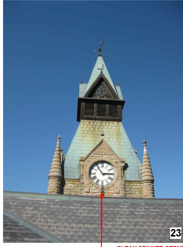
CLEAN STAINED STONE 23
