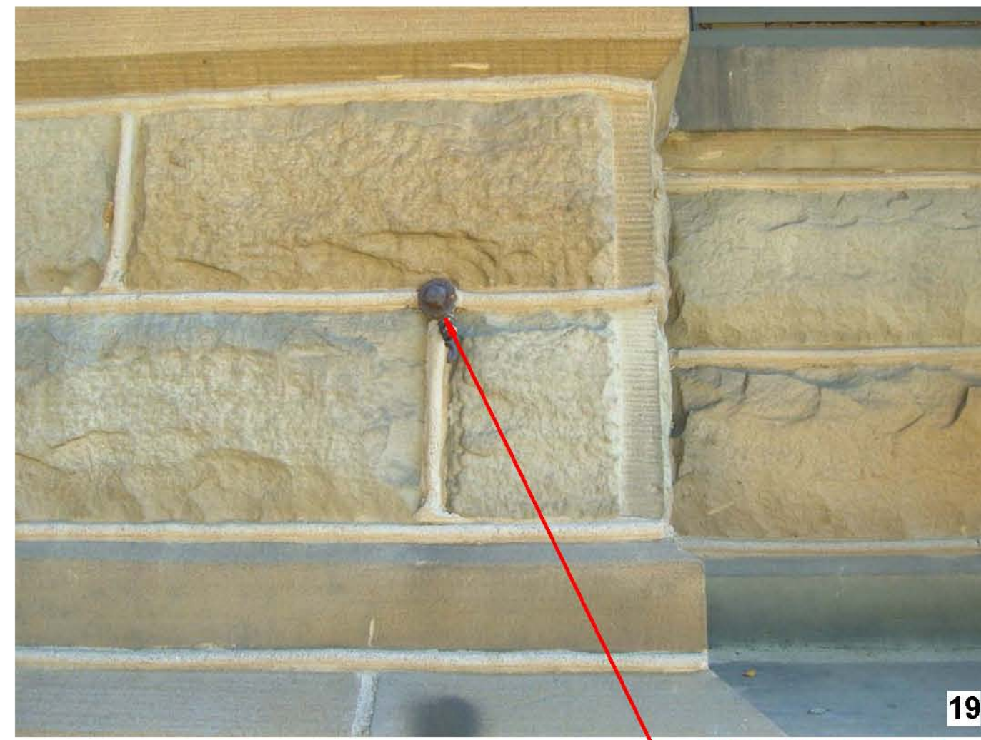
19 REMOVE BOLT, PATCH HOLE (STONE RESTORATION PACKAGE)
