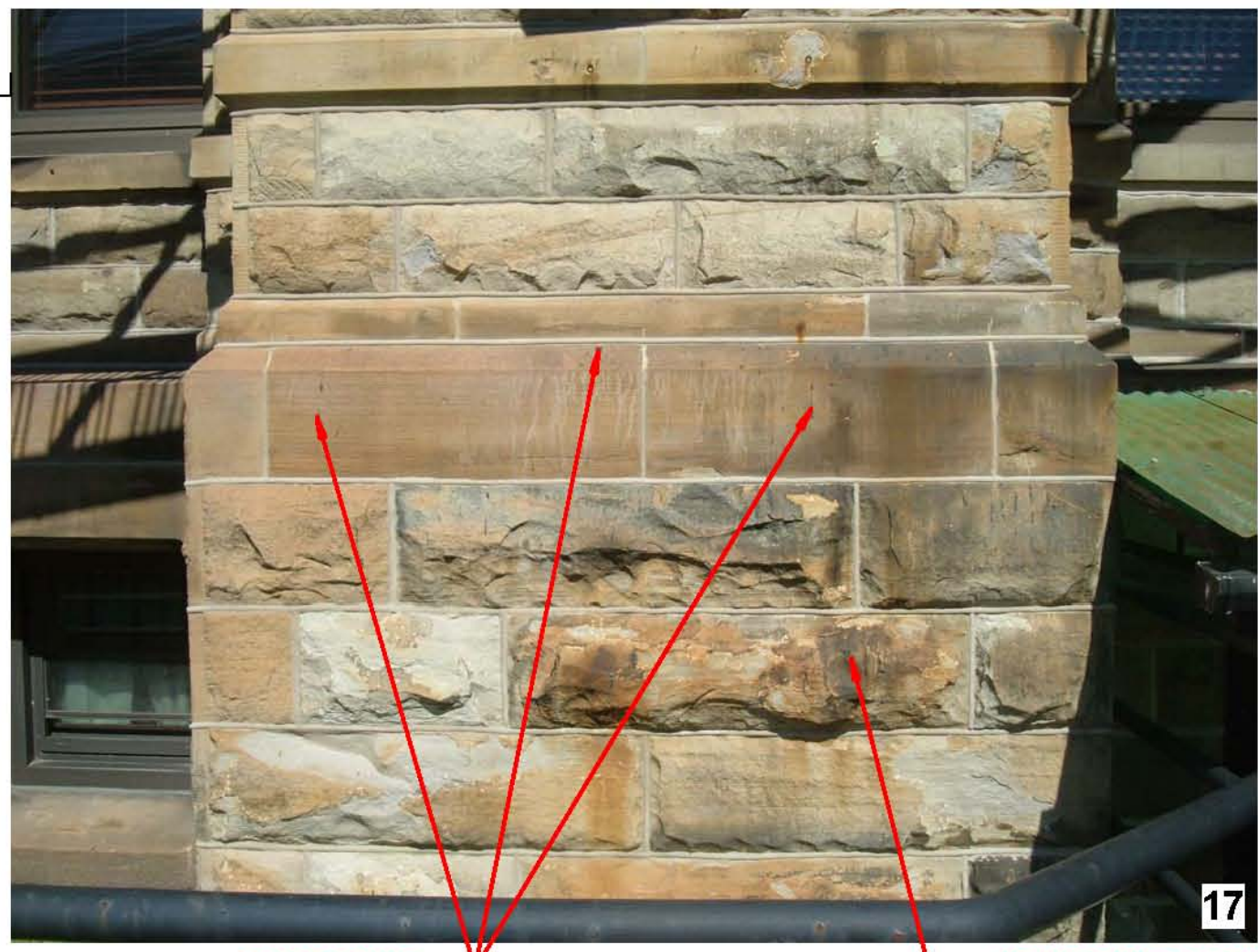
REMOVE PAINT CLEAN STAINED STONE 17
