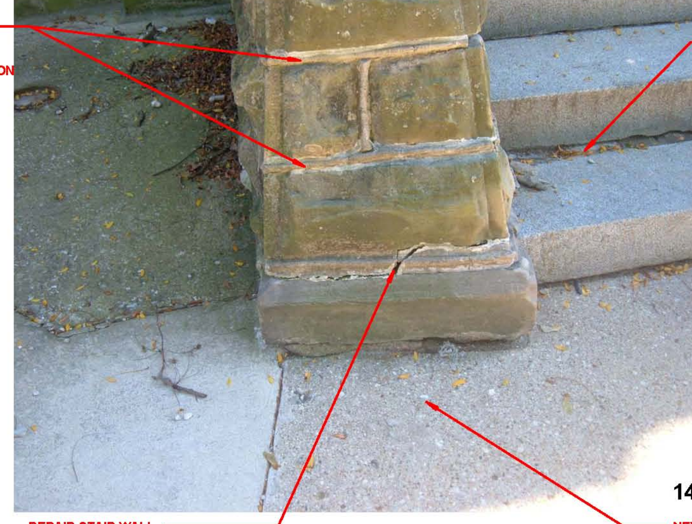
INSTALL BACKER ROD & SEALANT, TYPICAL @ ALL STEPS (STONE RESTORATION PACKAGE)
