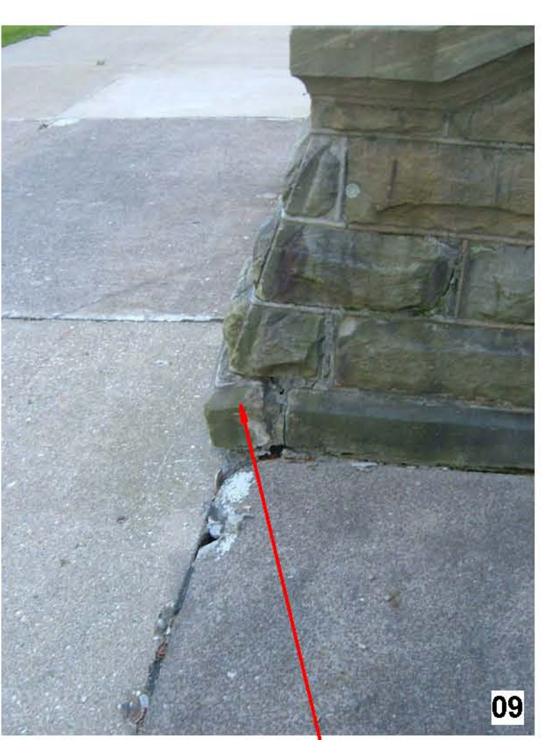
REPAIR STAIR WALL (STONE RESTORATION PACKAGE)
